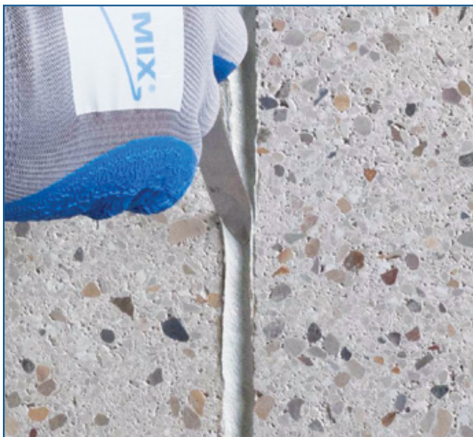
SPEC MIX SM100 Gray Sealant on an interior burnished CMU wall.
