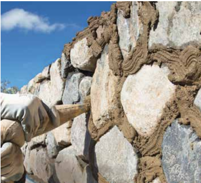
COLORED AVM USED IN JOINT GROUT APPLICATION
