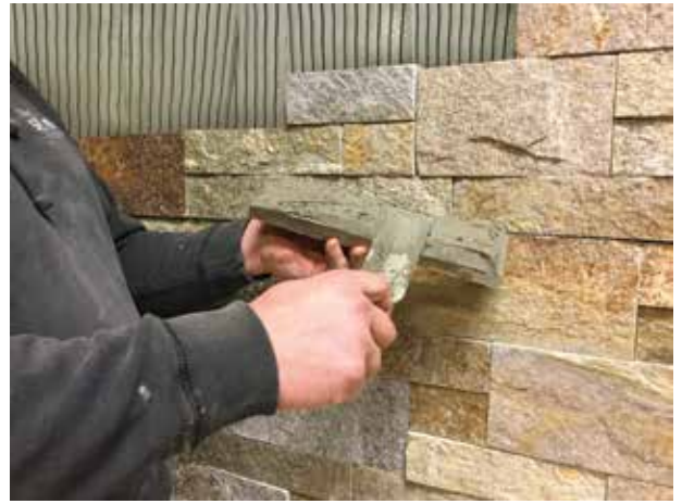
XP500 ADHESION MORTAR WITH NATURAL THIN STONE FOR BOND COAT APPLICATION
