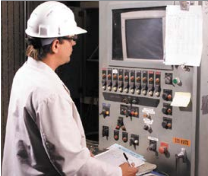
State-of-the-art batching for quality assurance
