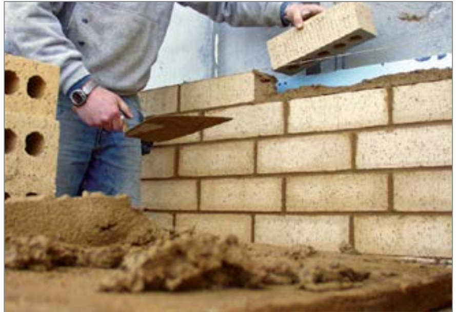
Consistent custom colored mortar, every time
