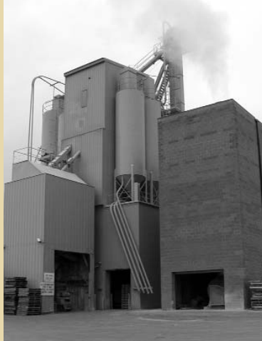
Twin City Concrete Product's St. Paul plant
