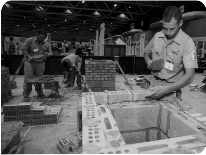
Joshua Hess lays another row of brick to his composite project in the National Masonry Competition held this past summer at Bartle Hall in Kansas City, Mo.
