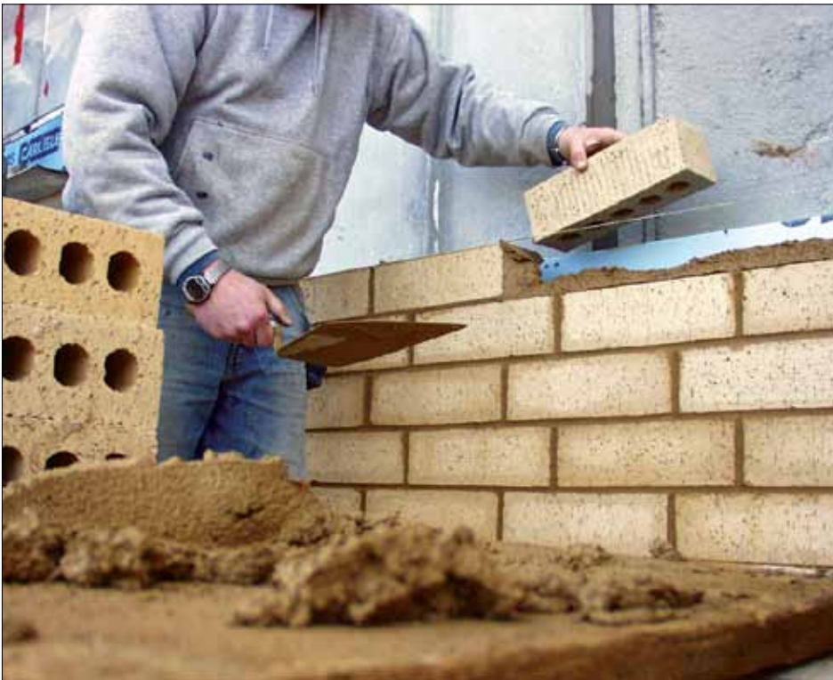
Consistent custom colored mortar, every time
