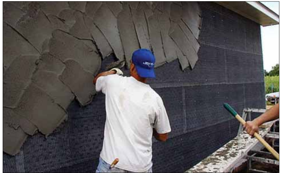
Application of proprietary, preblended, shrinkage compensated basecoat
