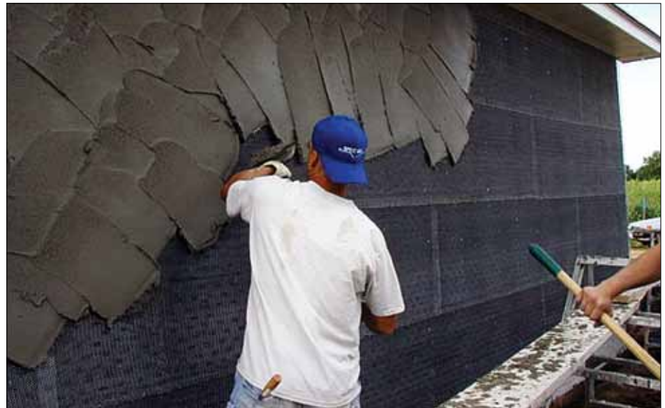
Application of proprietary, preblended, shrinkage compensated basecoat
