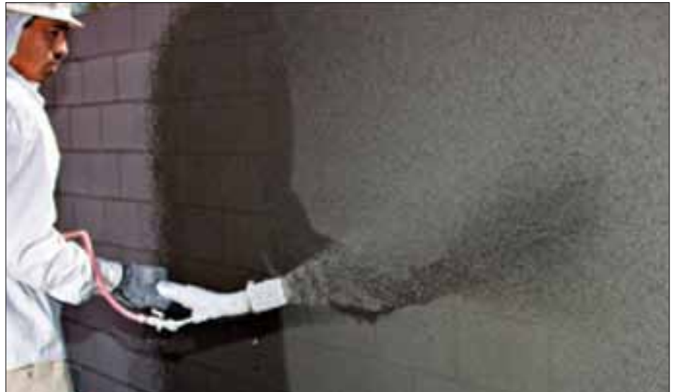
SPEC MIX FBC Stucco is engineered for gun-applied basecoat in one- and three-coat wall systems
