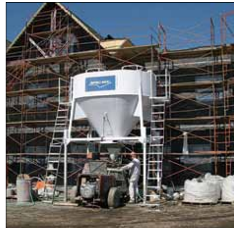
SPEC MIX silo system improves production and mix consistency and eliminates the disposal of wasted sand and bagged goods
