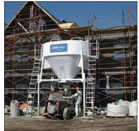
SPEC MIX silo system improves production and mix consistency and eliminates the disposal of wasted sand and bagged goods
