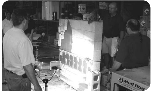
Left to right foreground; Mark Lukkarila/ SPEC MIX, and Stan Harwell/ SPEC MIX East Coast Sales Manager, observe Scott Ellingson/ TCCP-Iowa, pour the SCG into the test wall's core.
