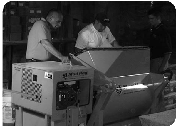
Left to right; Rolly Cox/ EZ Grout, Nick Blohowiak/ SPEC MIX Central Regional Sales Manager, Justin Meyer/ Midwest Block & Brick Sales Manager, mix the Ploymer Modified Stone Veneer in a new EZ Grout Mud Hog on-site for the crowd.
