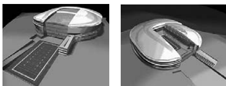
This will be the first stadium in North America to combine a retractable roof along with a mobile playing field. Upper Left: This view shows the playing field extended outside of the stadium on a mobile ramp system. Upper Right: This view shows the playing field retracted to the interior of the stadium.
