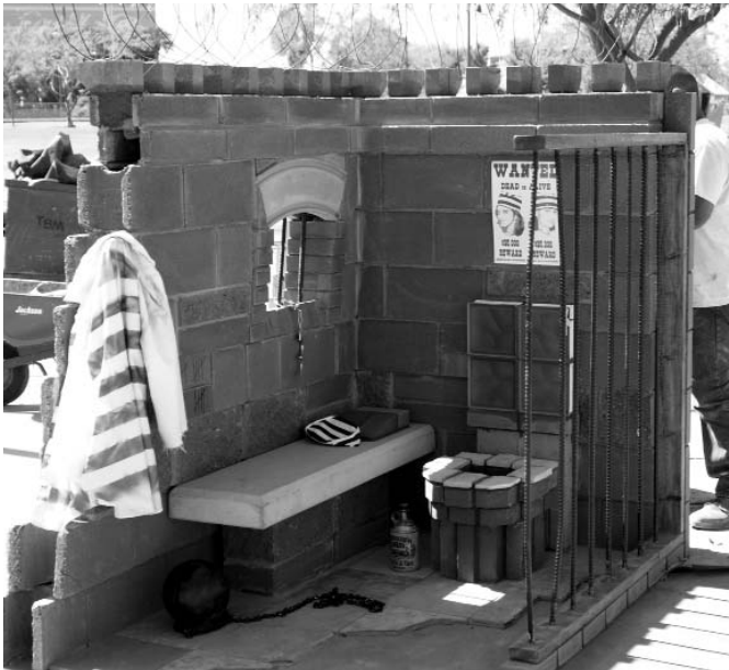
Architect and masonry team of Architectural Resource Team, Inc. and Sun Valley Masonry, Inc., take first place for their project titled “Jail” at the “Masonry: It Makes a Village” event in Tempe, Ariz.
